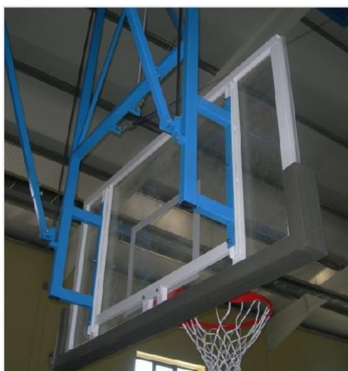
Fig. 2 Drop down goal support structure example
