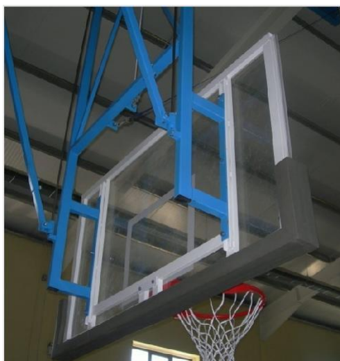
Fig. 2 Drop down goal support structure example
