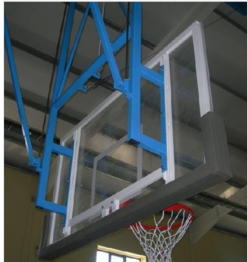
Fig. 2 Drop down goal support structure example
